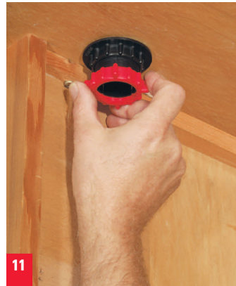
11. Carefully screw on the cone nut.
