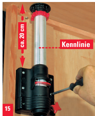
15. Tighten the screws. Leave 20 cm between the roof and the mounting bracket.
