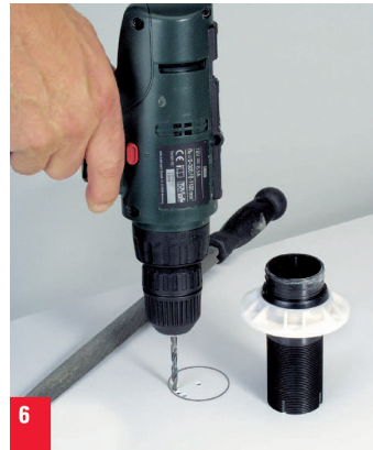
6. If you do not have a circular drill bit, draw a hole of \varnothing 38 mm for the roof duct and drill it out.
