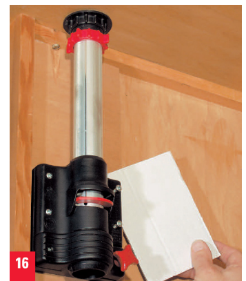
16. If it is difficult to move the mast, place an underlay underneath or sand it.
